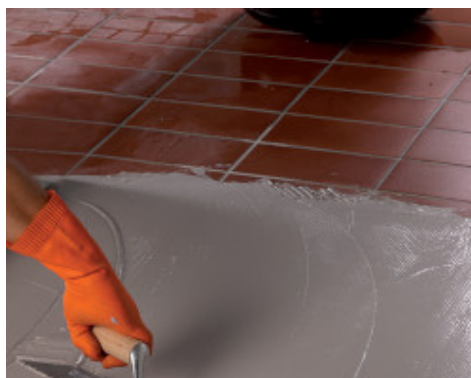
Applying a second layer of Monolastic on Mapenet 150
