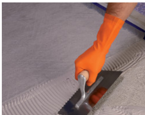
Applying a first layer of Monolastic welded with Mapetex Sel N on a new screed
